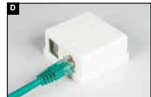
Snap the plug in place.
