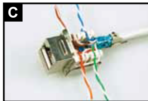
C Insert each wire into the appropriate channel according to the color code on the module.
