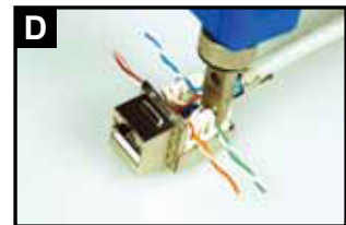
D Cut the surplus wires.
