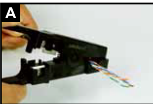
A Strip approximate 4cm of the cable jacket.
