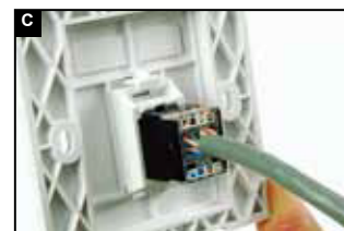
Align the jack to the slot.
