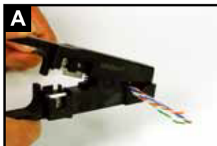
Strip approximate 4cm of the cable jacket.
