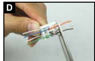
Cut the surplus wires.
