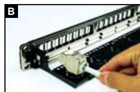
Position the shielded keystone jack after crimping.
