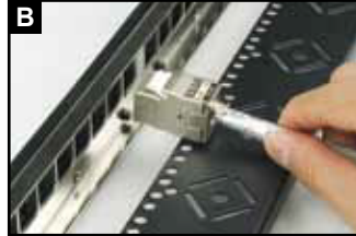
Position the shielded keystone jack for installation.
