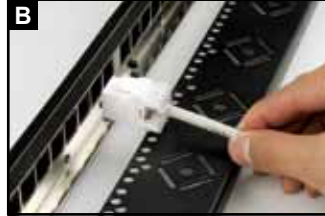
Position the shielded keystone jack for installation.
