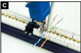
Terminate wires using Linkbasic tool or equivalent.
